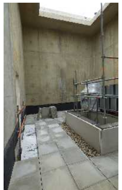
7. Top of the Tower Internal
